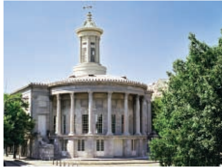
14 Merchants' Exchange 3rd Street at Walnut Street 215.597.8974
